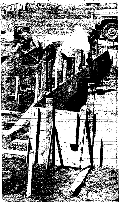
CONSTRUCTION is underway near the Bill Moore residence in Dixon of a new fur trading post. The building will house machines to skin animals as well as office space to conduct business in a four state area. Working on the project is Bill Sr., left, and his son, Bill Jr.
